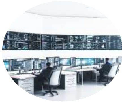
Integrated emergency command center
